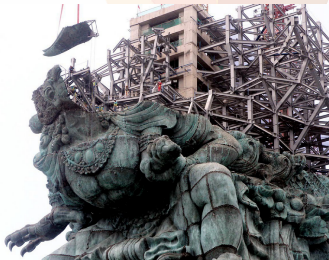
Figure 2. Supporting steel framework and installation of the GWK "skin" Source: Nuart Sculpture Park archives
