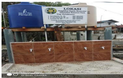
Figure 7. Installation of water faucets
