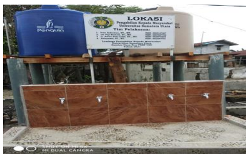
Figure 7. Installation of water faucets
