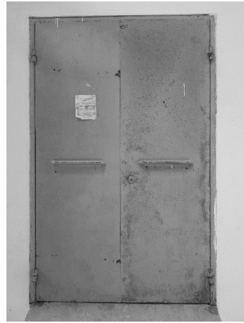
Gambar 12 Pintu loading dock
