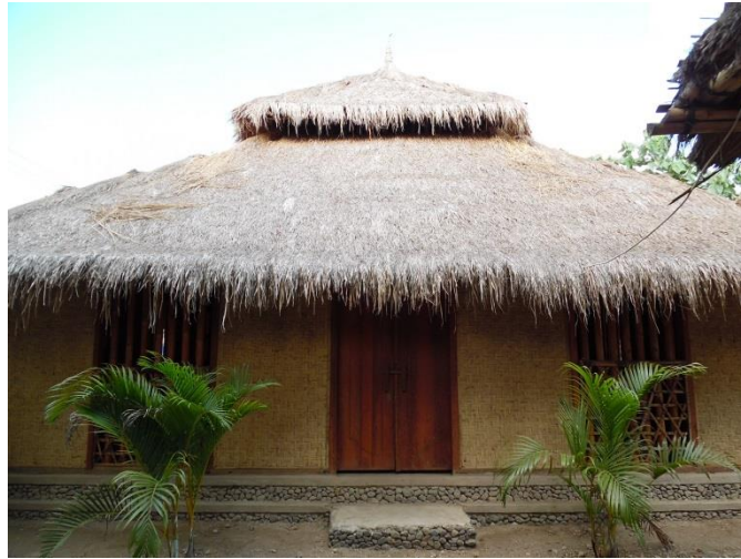
Picture 1 Traditional House in Sade Village (Source: Researcher Documentation)
